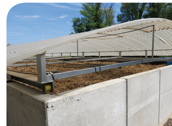
Concrete side and rollable roof
