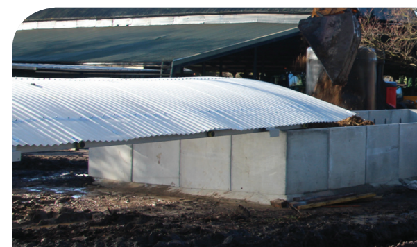
Concrete panel construction with rollable roof
