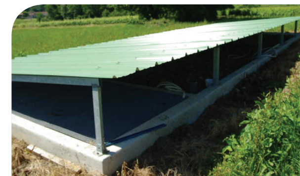
Below ground construction with coated steel roof
