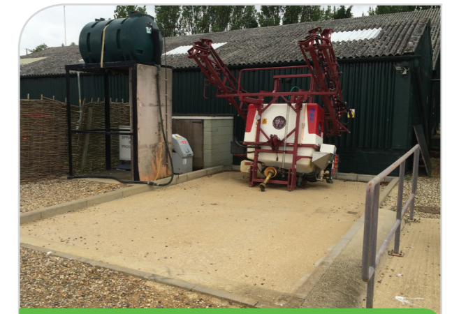
Good sprayer fill site. Good control by bunding and separate drainage to a biobed
