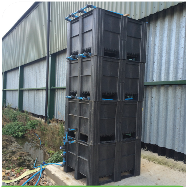
Stacked biofilter from a covered sprayer fill area
