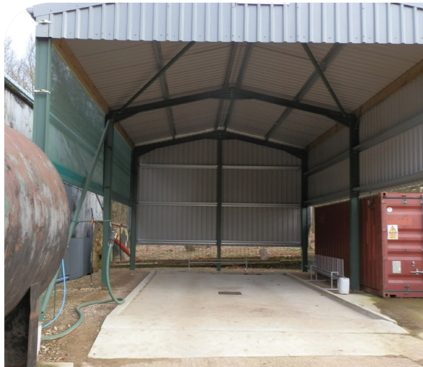
Roofed fill area, controlling rainwater inputs, well bunded containment of inadvertent spills and drips
