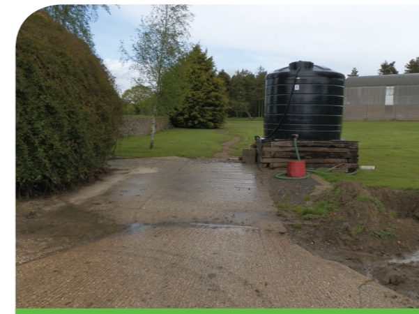
Poor sprayer fill site. Cracked sloping concrete, no control of liquids spilt
